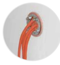
Drilling for cable passage PEXTBALI
