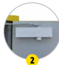
2 Self-closing door with thermo-fuse
