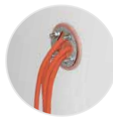
Drilling for cable passage PEXTBALI
